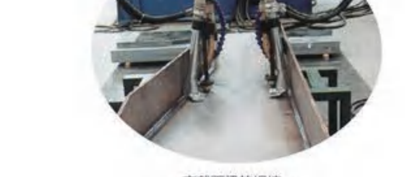
变截面H型钢的焊接 Welding of the Variable Section Beam
