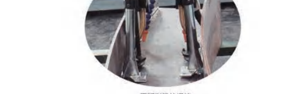
固定截面H型钢的焊接 Welding of the Fixed-section Beam
